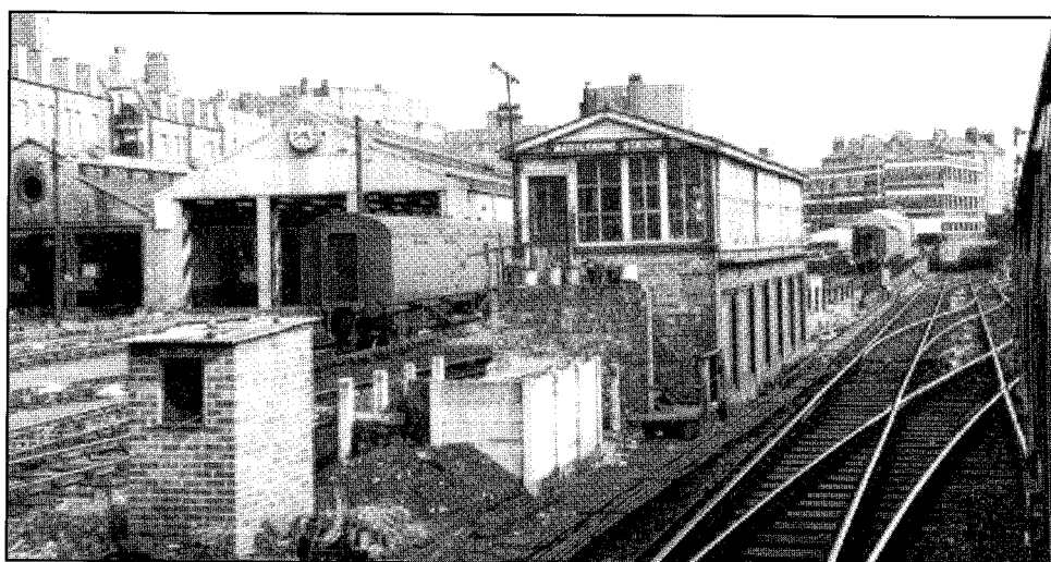
Marylebone Station Signal Box in the 60's. Note the easily recognised Great Central architecture of the shed to the left of the carriage shed. GCRS Collection.
